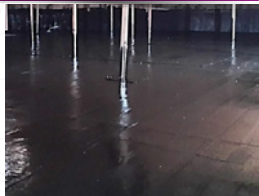
▲ Petroleum storage tank after reinforcement by laminated composites
