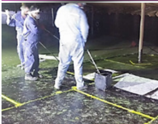
▲ The implementation of composite coatings on the floor of a corroded tank
