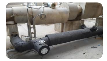
Refrigerant cycle vapor recover's position to boil-off gas compressor's suction of propane's storage in order to recovery of propane's vapor to control pressure of refrigerant cycle.
